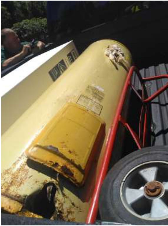
Replacement of old 1989 Water heater in the Satellite Bath!
