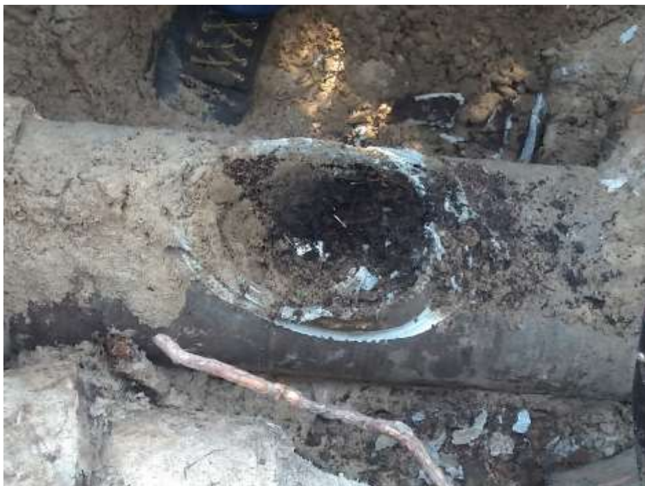
RECENT SEWER REPAIR ON SAILER LANE.
