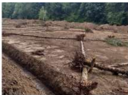
Step 3: Install Log Maze, release stream and replant.
